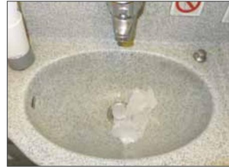
Improper use is often the reason for a blocked drain. Hand towels into the toilet bowl or sink can easily block a vacuum toilet or a sensitive wastewater piping system. And "young minds" have often felt the need to conduct experiments by dumping tissue down often very old drainage systems just for fun!
